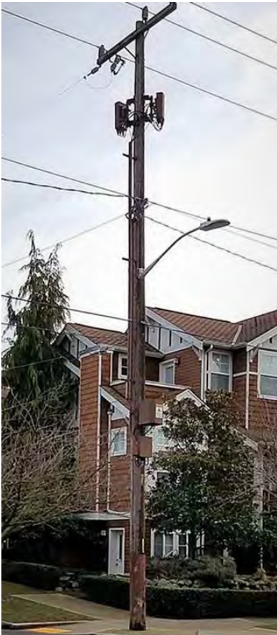
Typical wood pole design with panel antennas
